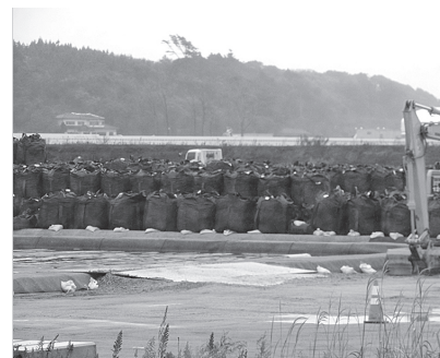
Piles of black flexible containers filled with contaminated soil from cleanup operation
